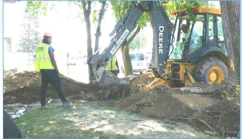
* Lead Service Line replacement (Flint)
