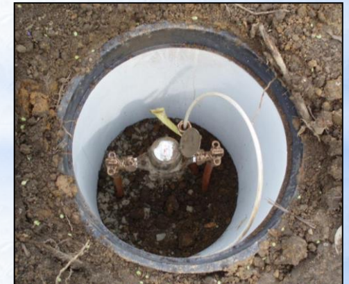
* Neofit Installation (Louisville)
