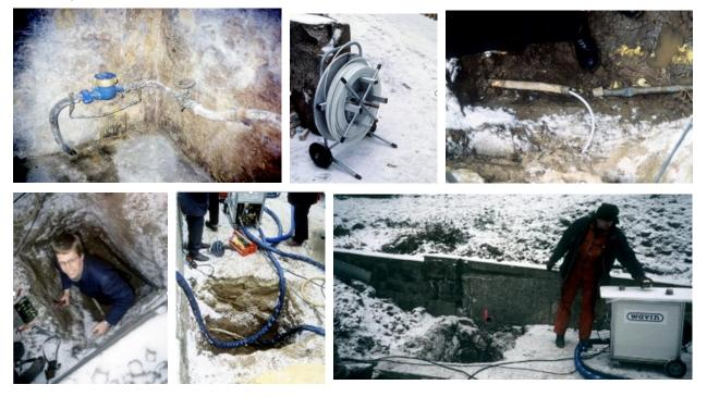
As per date of this report (23 yrs later) the with Neofit lined lead service pipe is still in operation, with very satisfactory performance, supplying 140-160 m<sup>3</sup>/yr.
