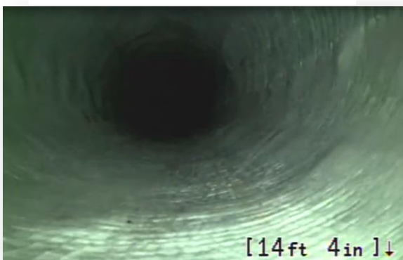
After Flow-Liner® was installed
